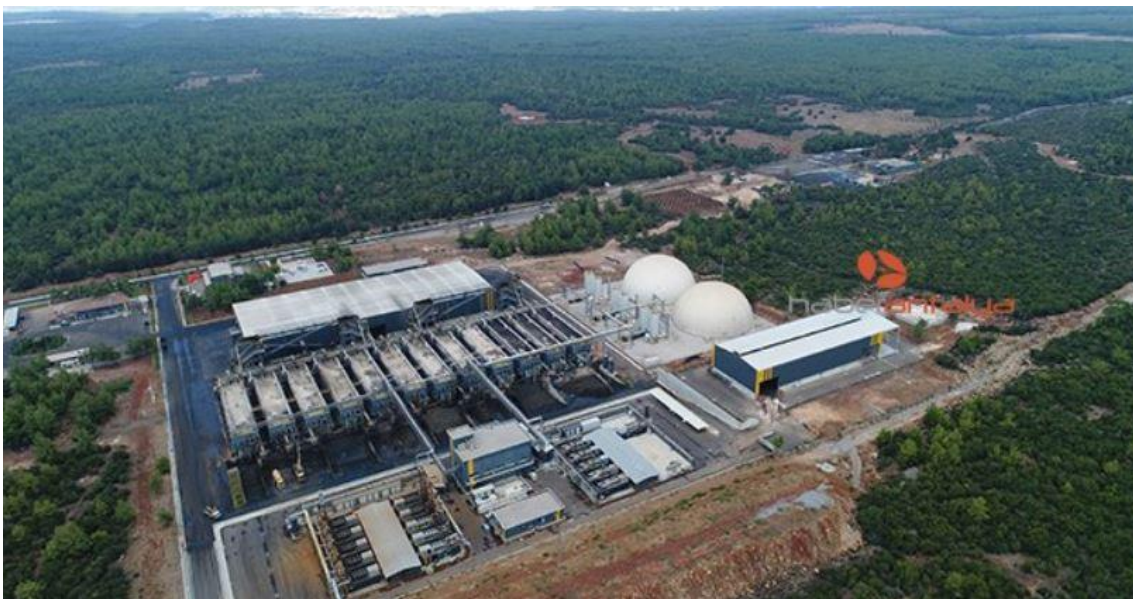
Figure 7 Aerial view of Antalya Kızıllı Waste to Power project
