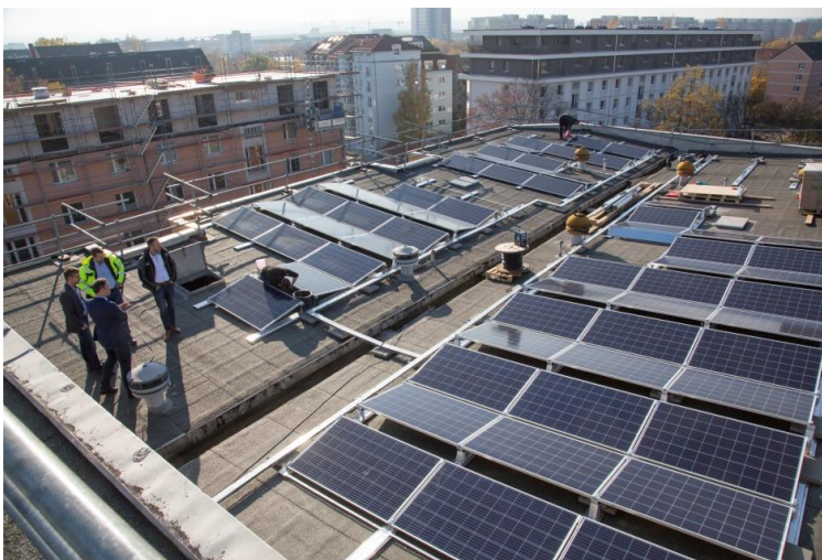
Figure 50: Photo of the construction process of the photovoltaic system
