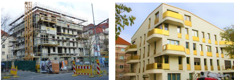
Figure 26: Unfinished construction in 02/2018 (left) & finished house in 09/2018 (right)
