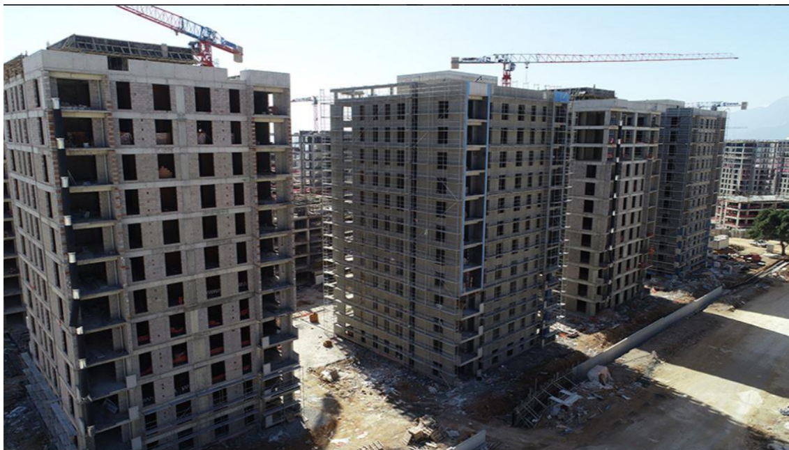
Figure 9 Construction of buildings
