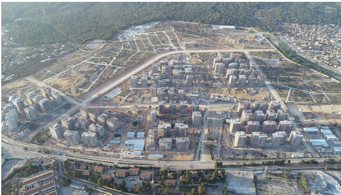
Kepez Santral Regeneration Project during construction
